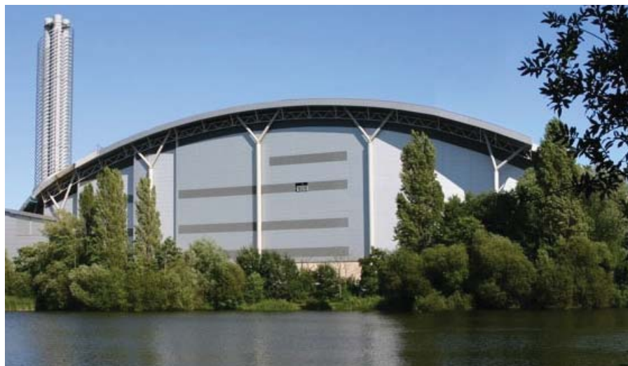
The Lakeside Energy from Waste facility in the UK can process 410,000 tons of waste per year, generating 37MW of electricity (enough to power 50,000 homes). As of this writing, the company that built and manages this facility was one of the top ten holdings of the Green Century Balanced Fund (see p. 6).
